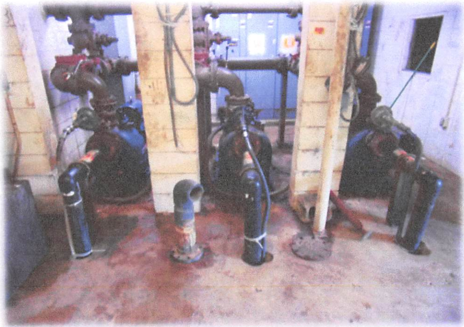
Wastewater main lift
